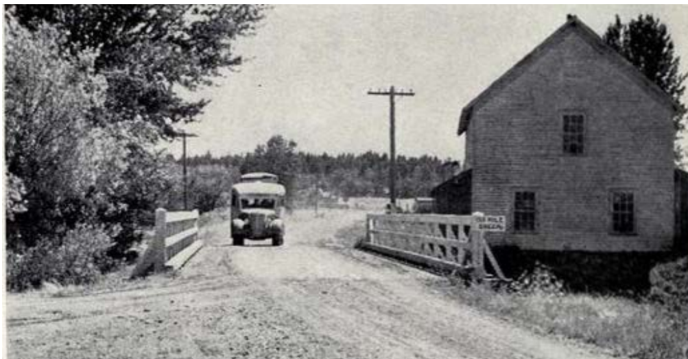
Cariboo Waggon Road at 150 Mile Creek, 1946
