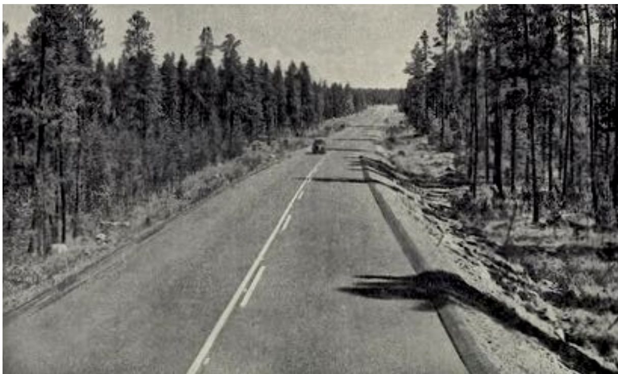
1950: Newly constructed and paved Highway 97
