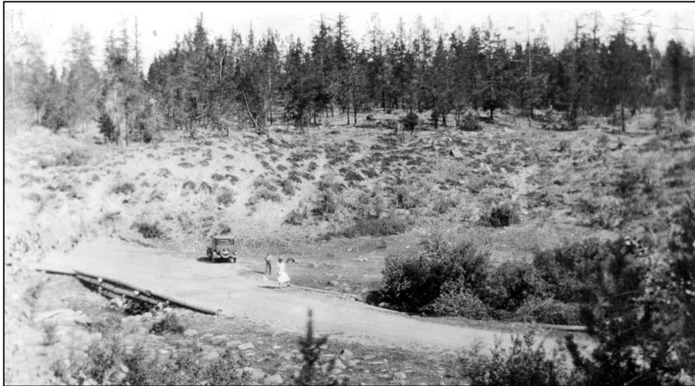
The CWR as it crossed 57 Mile Creek at junction to Chasm. Today the creek runs underneath the highway
