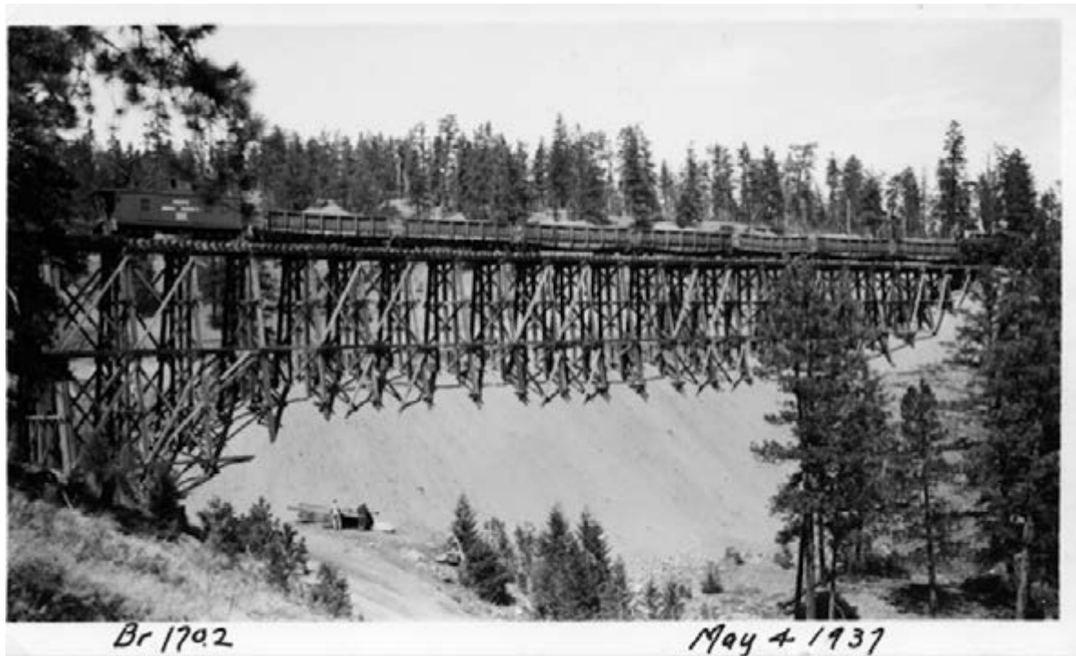
Railway trestle at 51 Mile as it appeared in 1937; it is now completely filled in. This was done routinely as it was much cheaper than rebuilding aging trestles
