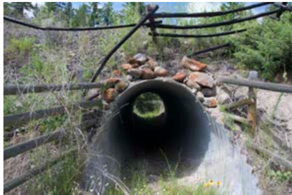
Large culvert: future plans include new fencing and a gate
